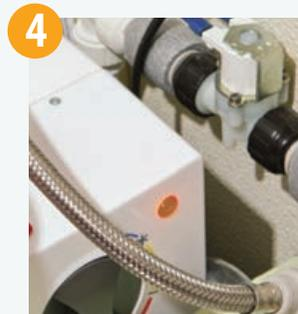
Check to see if the amber LED light on the water heater is illuminated, if not then it may be the 13amp fuse in the switched spur which requires changing.
