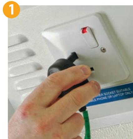
1. Remove the appliance from the inverter powered socket
