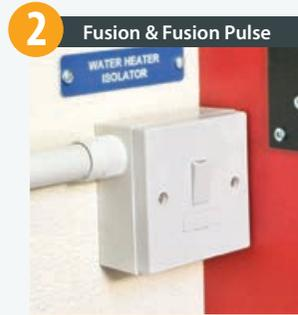
Ensure the switched spur for water heater is in the 'ON' position.
