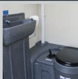
Toilet wash area
