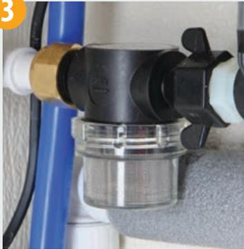
Check inline filter for any visual signs of leakage or damage to casing.
