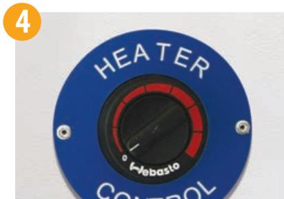
4 Return to the control panel in the canteen and turn heater control anti clockwise to the "off" position.
