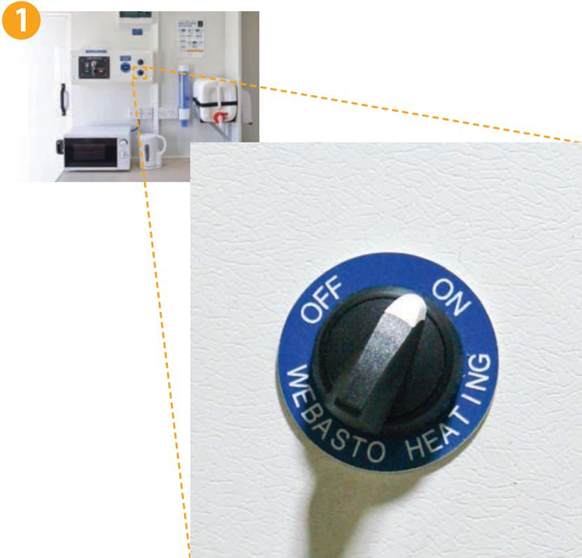
Turn the heater control toggle switch, situated on the control panel in the canteen, clockwise to the "ON" position.
